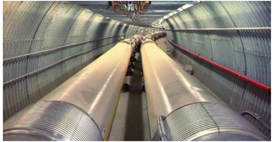
New equipment will be added to these giant, underground tubes used to isolate and test molecules, leading to research that could involve up to 1,000 scientists from 30 nations.
